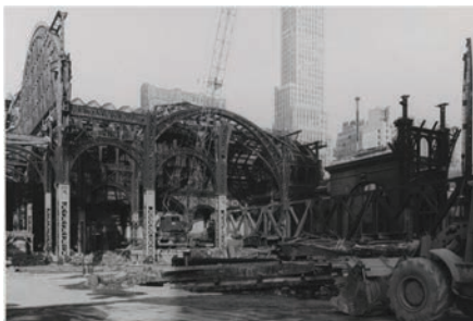
Penn Station being demolished.
