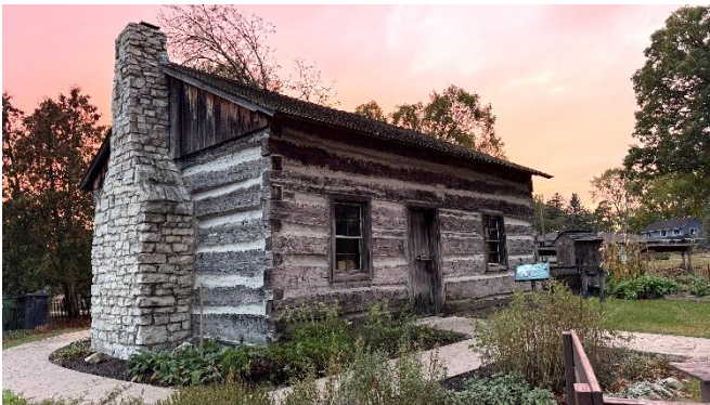
Relocating the Log Cabin will be the first and most important part of the West End Expansion Project. Slated for next spring and summer, it will improve the flow of the Village and enable us to incorporate currently underutilized spaces.
